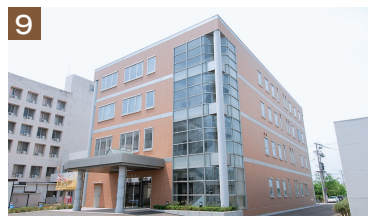
9 School of Nursing Building (offices, lounge, meeting rooms, lecture rooms, labs)
